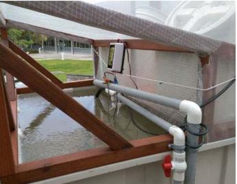
The solar system utilizes two 12v, 50 watt panels, mounted at a 90 degree angle to each other, and oriented south. The panels are slightly over sized for the power required so that during overcast days, the system can still operate normally. The eastern rising sun to strikes the first panel at sufficient angle to
